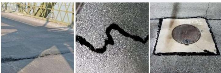
**SigilRapid Plus** is a cold, single-component, elastic, polymeric sealant, ideal for sealing surface cracks on bituminous and concrete floors. It has been specifically designed for manual casting with rapid surface cross-linking. Certified for airport floorings.
