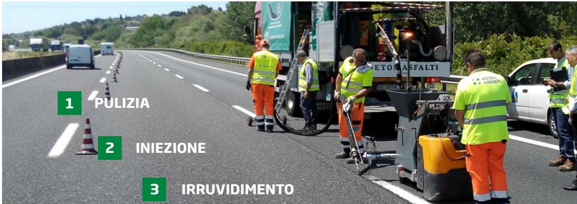
**SBS Sigil PLUS** is a technology that uses a mobile plant for its installation that is unique and complete with all the professional equipment needed for the execution of hot-sealing and longitudinal and transverse road surface cracks, guaranteeing a high level of productivity, rapid execution of construction sites, easy movement and total independence.
